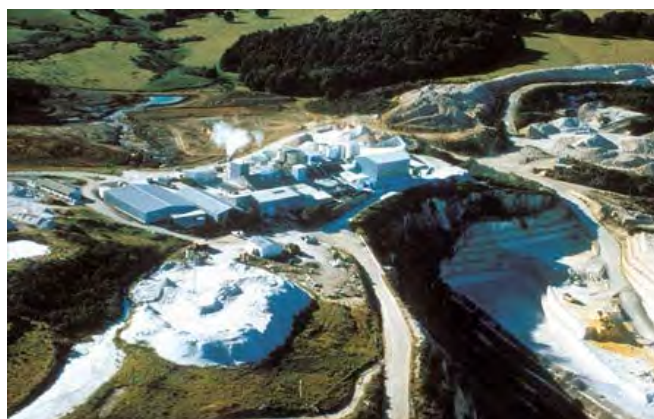
Figure 53. Matauri Bay clay pit
